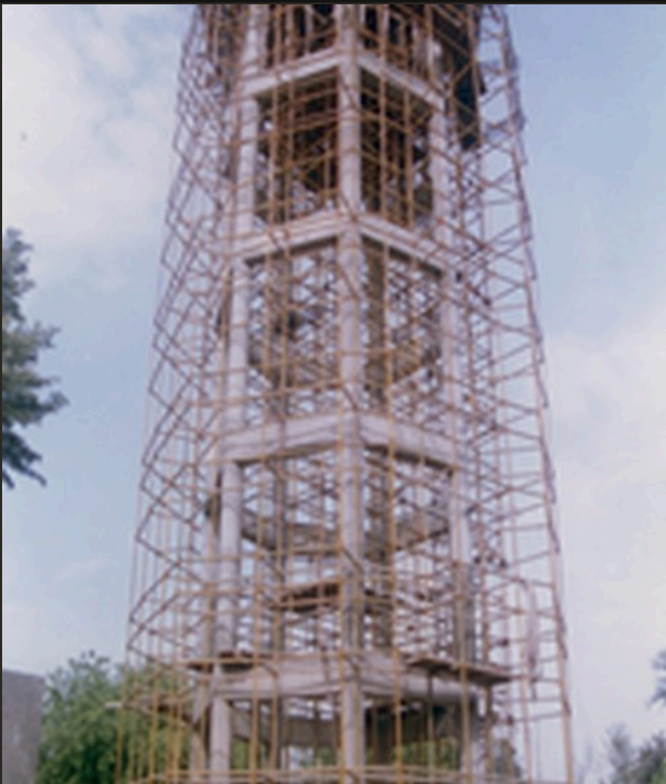
IFFCO Water Tank, Sector 17B, Gurgaon
