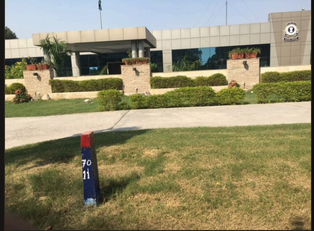
Completed campus works
