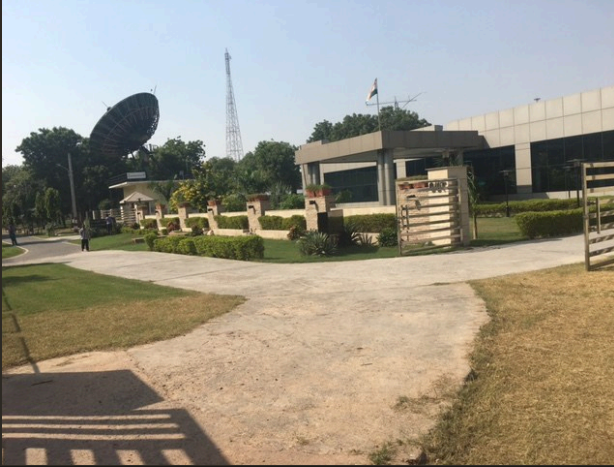
Completed campus works
